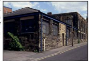
Former Springwell Brewery premises in Church Street, Heckmondwike, May 1993.
